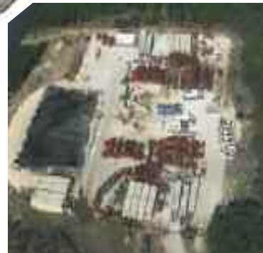
Figure 5 – Example of fracturing operations, aerial view
