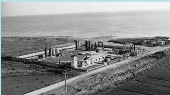
First gas treatment terminal in Europe
